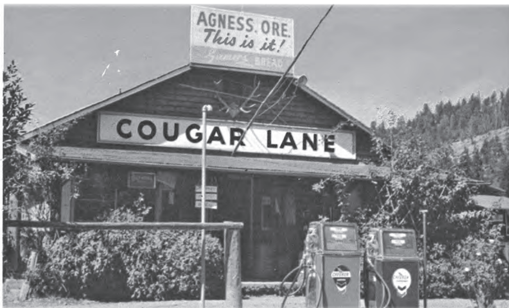
Cougar Lane store after power line was built (Photo courtesy of CHS)
