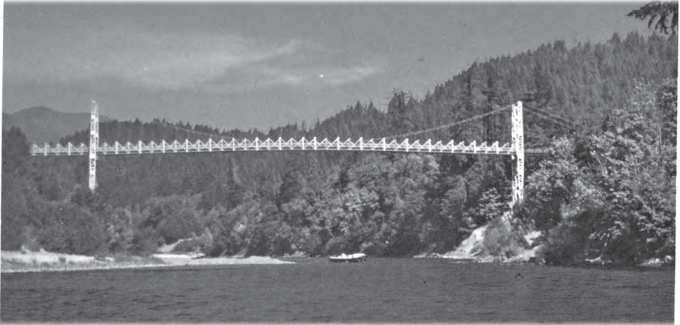
Suspension bridge in Agness (Photo courtesy of CHS)
