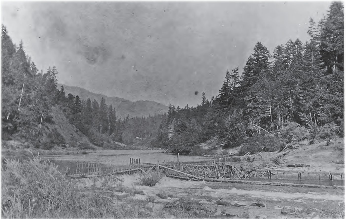
A wing dam on the Rogue River between Agness and Illahe at the Old Diggins Riffle. Circa 1912. House in center is the Price home, white on tree to right of center was an old shag roost, white gravel on left are tailings from Gold Bar Placer Mine.
