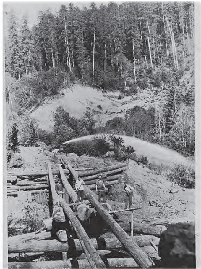
Bridge to Camp Inman Mine
